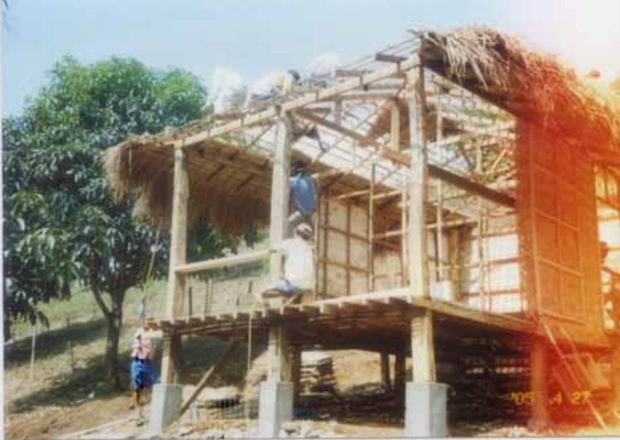
COGON GRASS IN BUNDLES SERVES AS THE ROOF
